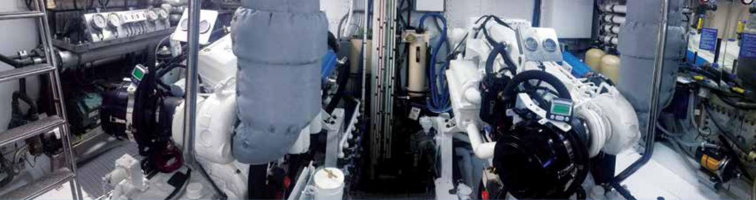
The engines were bolted straight onto the existing gearboxes, says First Mate Graham Jones.
